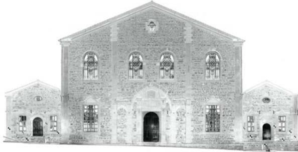
Figure 5. Facades produced by 3D laser scanning model
