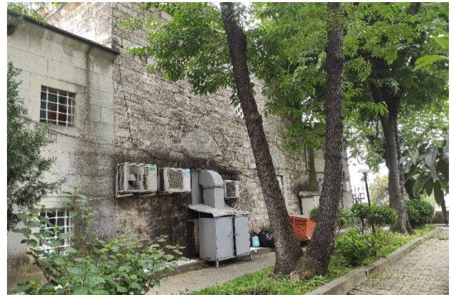
Figure 9. The external wall of the classroom showing the incompatible fittings and poor maintenance of the historic fabric, 2021
